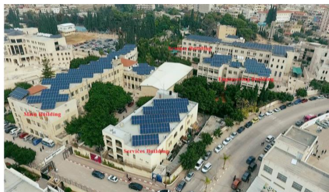
Figure (2): PV installed systems on roof tops of some of PTUK buildings.
